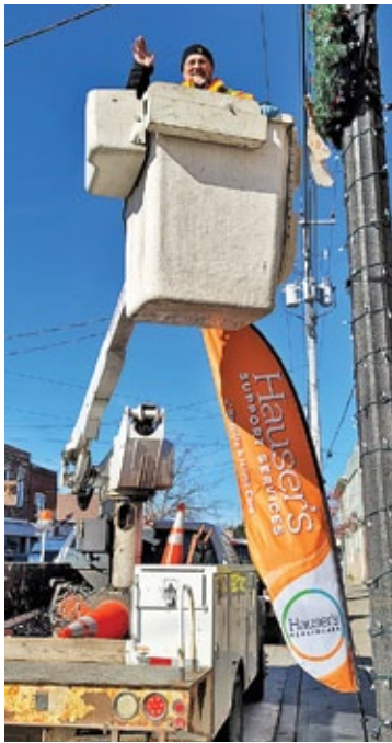
A bucket truck from Norfolk-Simcoe Electric helped take down the old lights and install the new strands.
