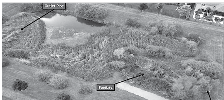
Today the pond on Angler Avenue is choked with sediment and vegetation. Photos from county report
